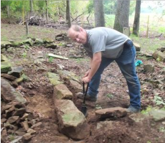
Scott Giltner repairing an old stone wall at Old Livingston Presbyterian Cemetery near Fredonia, KY. Two Rev. War Soldiers are buried in the cemetery.
