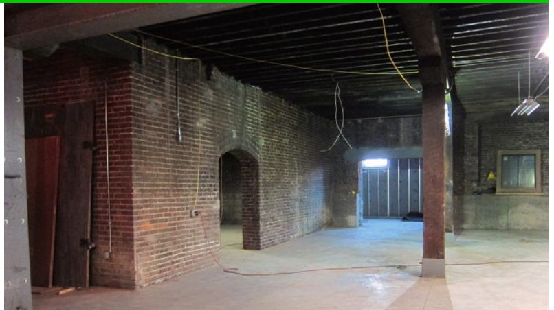
Pictures of Basement
